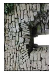
STONE HEAD EAST WINDOW FAILING SOUTHERN REVEAL COLLAPSED
