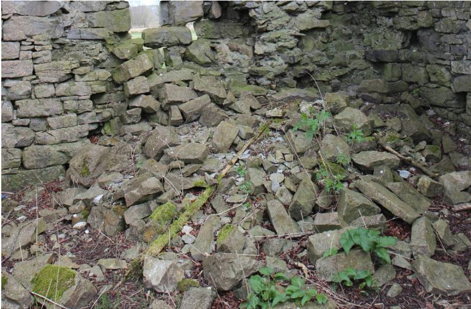
**Photograph 8 Fallen Stone from Inner Face of East gable**
