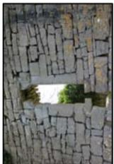
DRESSED STONES FROM OUTER ELEVATION CRACKING AROUND OPENING DUE TO STRUCTURAL FAILURE
