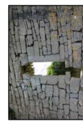
DRESSED STONES FROM OUTER ELEVATION CRACKING AROUND OPENING DUE TO STRUCTURAL FAILURE
