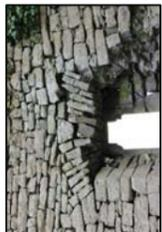
STONE HEAD EAST WINDOW FAILING SOUTHERN REVEAL COLLAPSED
